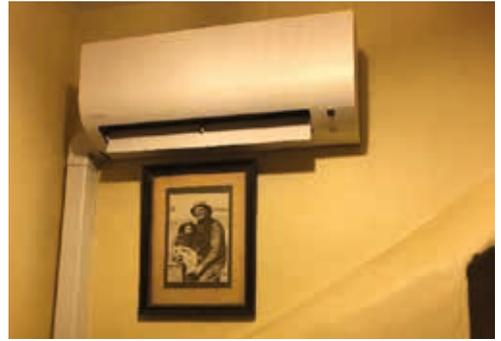
If the property is listed, Listed Building Consent will be required. The visual impact of the heat pump will need to be considered, and whether it could be removed without damaging the building. It may be approved if positioned in a visually discreet location on the rear elevation and without extensive invasive works to the fabric of the listed building.
