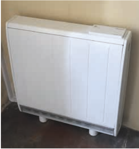
New high heat retention storage heater
