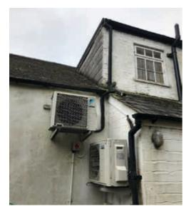
Above and top right: Images of external unit and internal air to air heat pump
